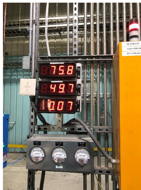
Figure 6: Booth Monitoring Stack Showing 75.8°F and 49.7% RH
